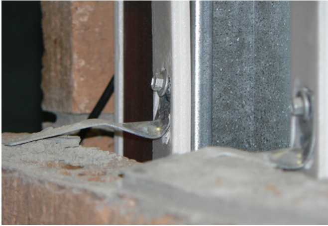
Permanent deformation of brick ties at end of tests.
