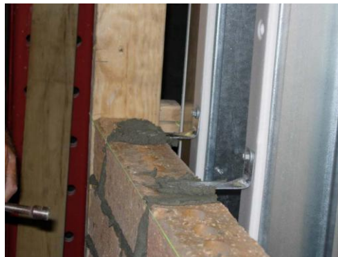
Tie fixed to thermal break (Wrap emitted for clarity)
