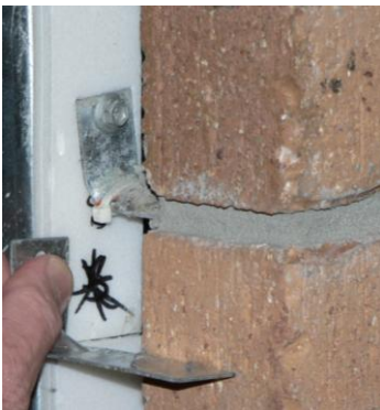
Tie fixed to thermal break (Wrap emitted for clarity)
