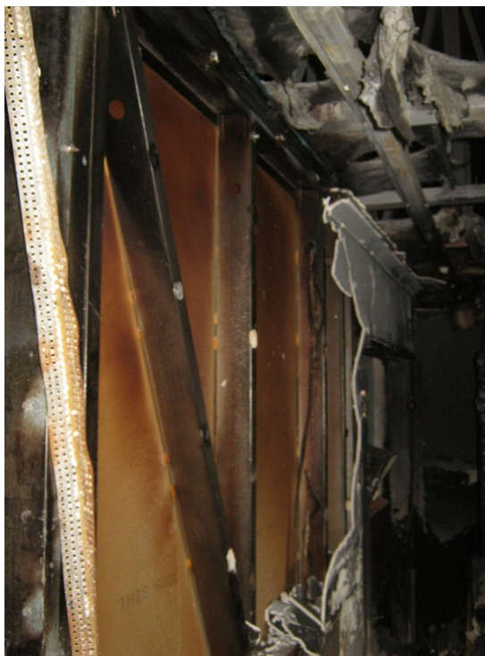
Figure 15: Undistorted steel framing in the walls
