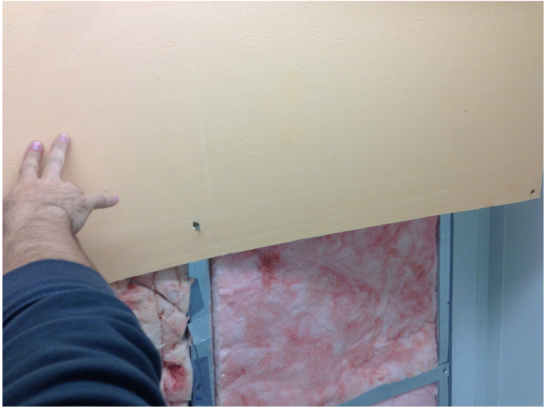
Figure B9. Eighth day check (Completely dry)
